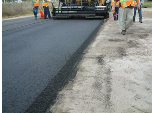
Paving road with safety edge
