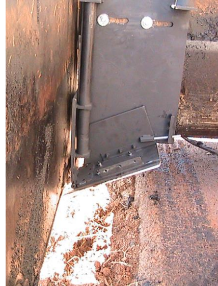
Unit Attached to Screed Extension with Gap between End Gate
