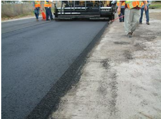
Paving Road with Safety Edge
